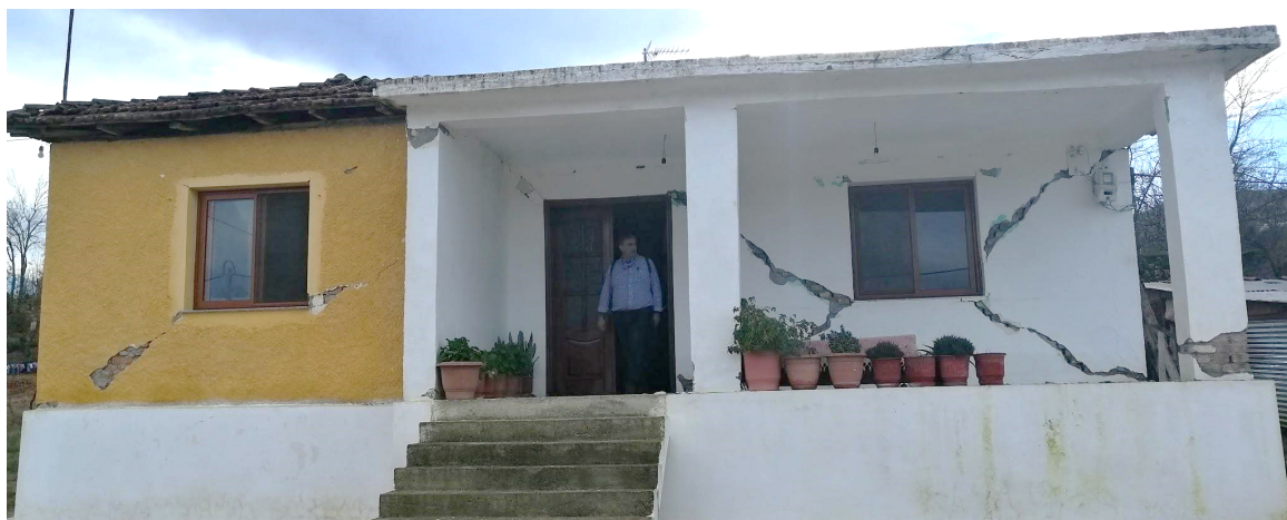
Figure 28: Moderate damage of single-storey building in Thumanë
