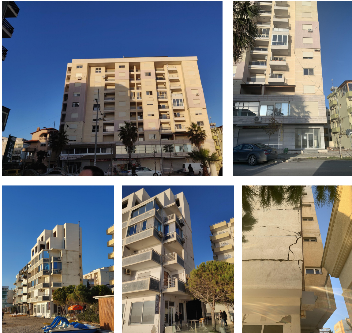
Figure 25: Light damage at hotels in Durrës
