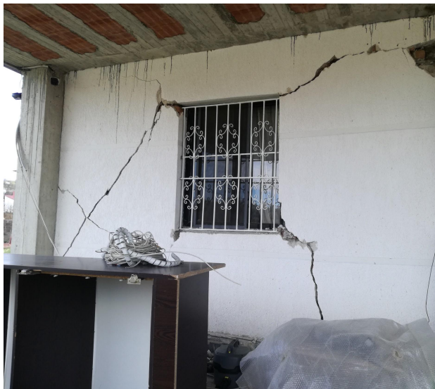
Figure 35: Moderate damage of two-storey masonry building with stone bricks, extended in plan with RC frames in Thumanë.
