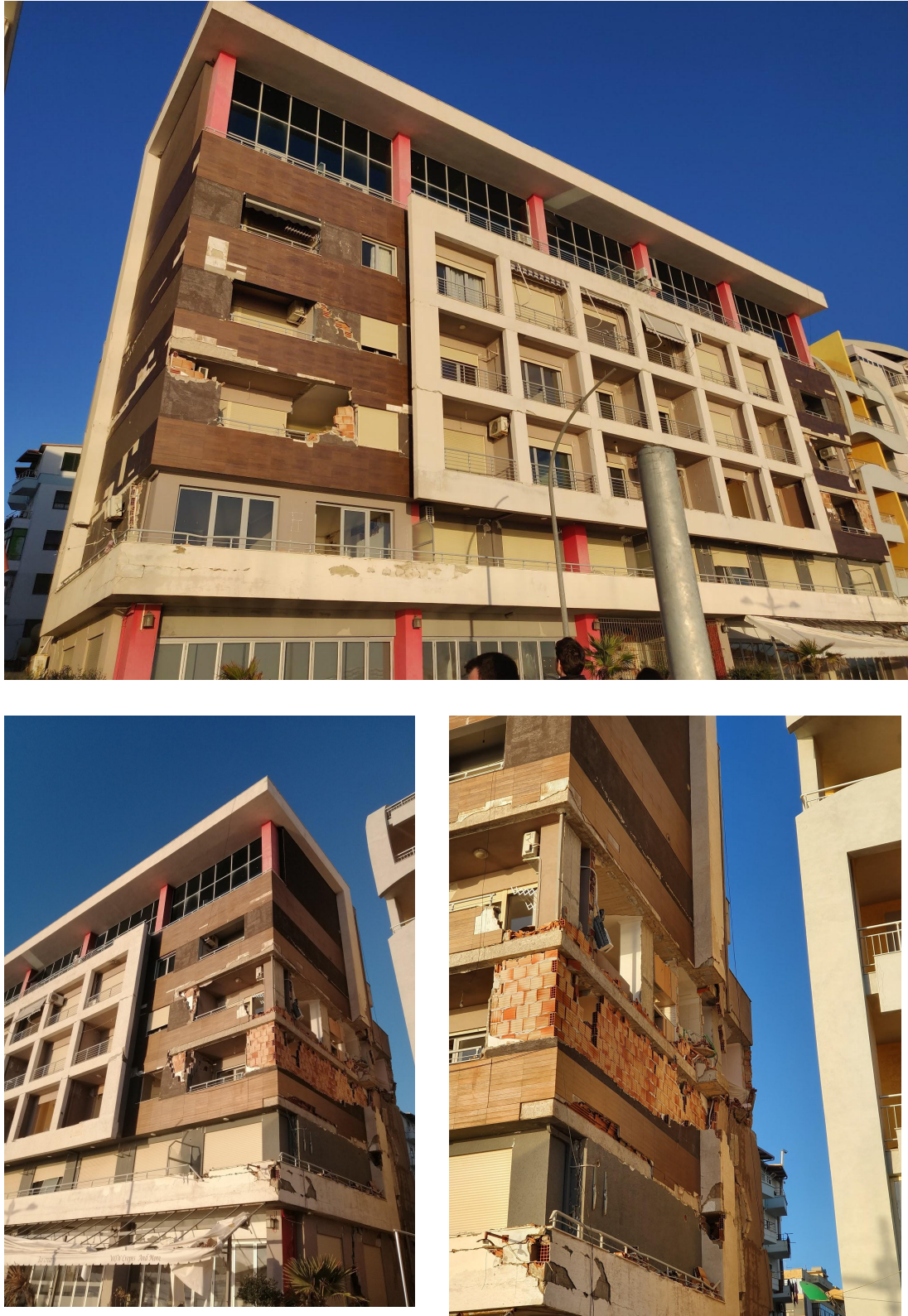
Figure 19: Major damage of a 5-storey RC building. No confinement of the brick masonry walls to the RC frame is observed.
