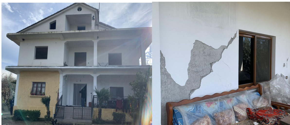
Figure 30: Moderate damage of three-storey building in Thumanë
