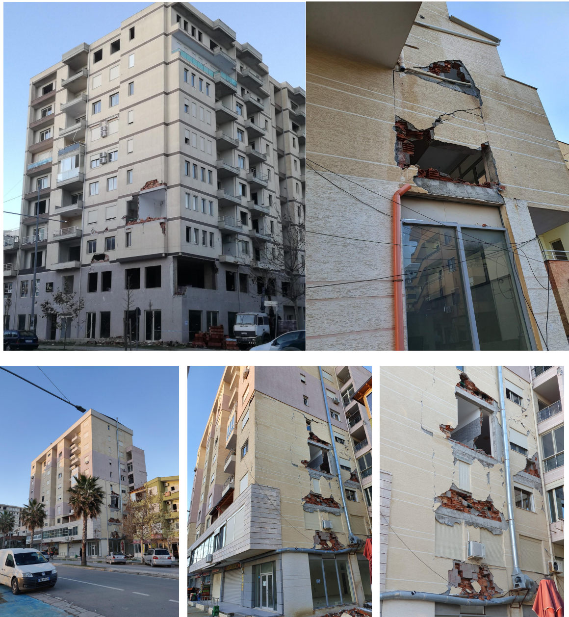
Figure 21: Major damage of a 10-storey RC building.
