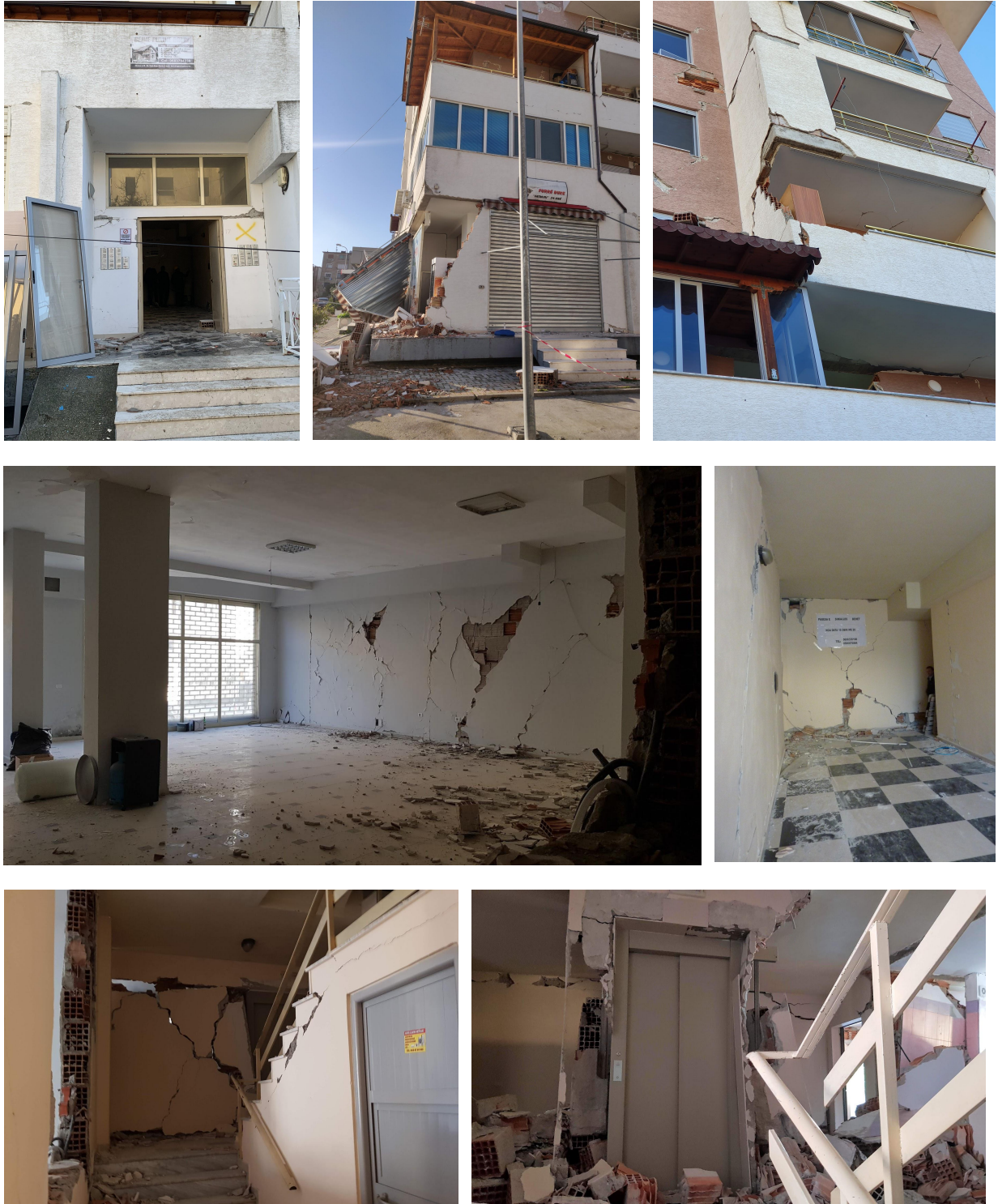
Figure 20: Major damage of a 6-storey RC building (continued).
