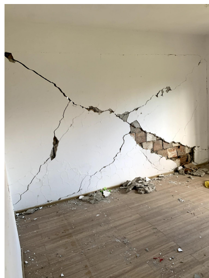
Figure 36: Major damage of two-storey RC building in Thumanë
