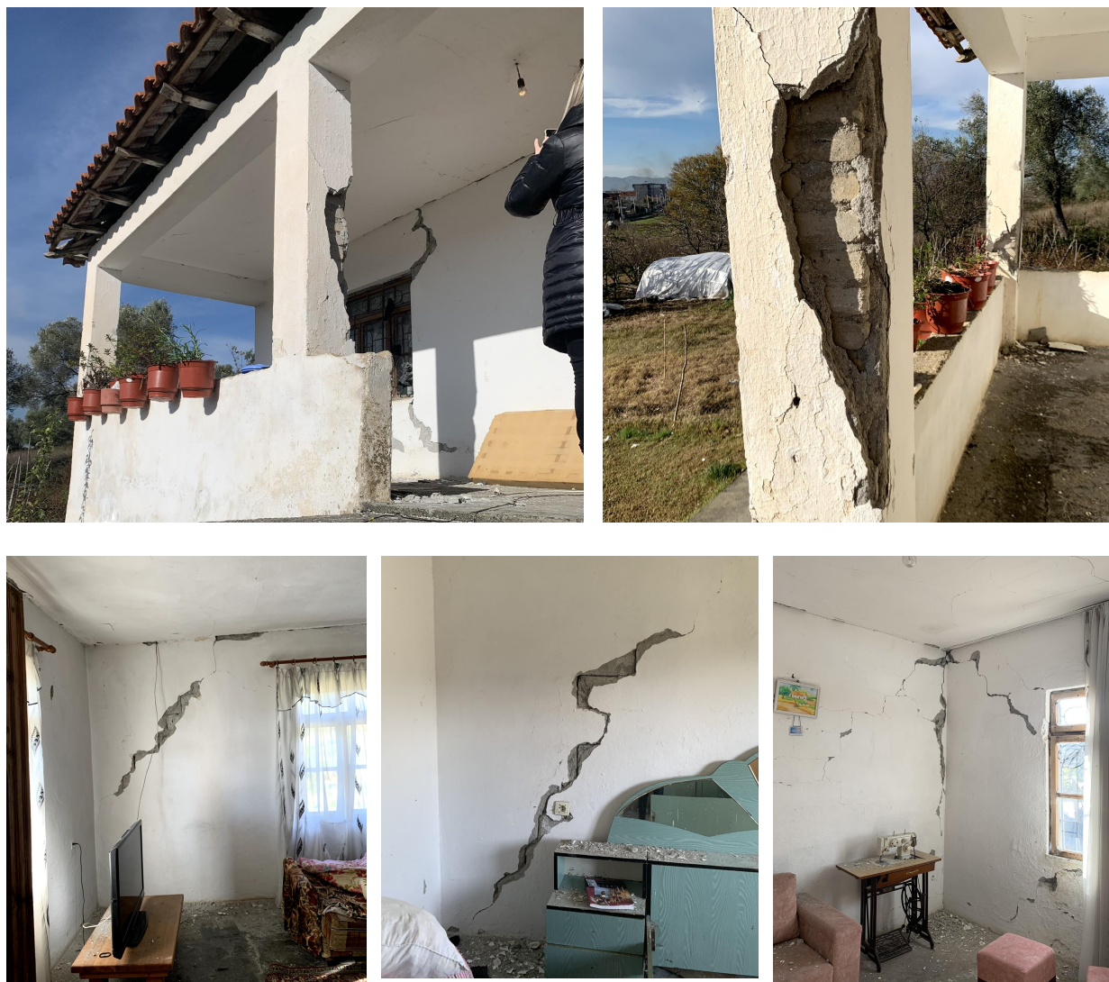
Figure 38: Major damage of single-storey building in Thumanë
