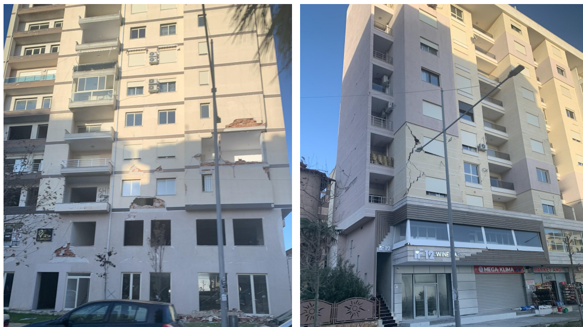
Figure 15. Moderate damage of a 7-storey RC building
