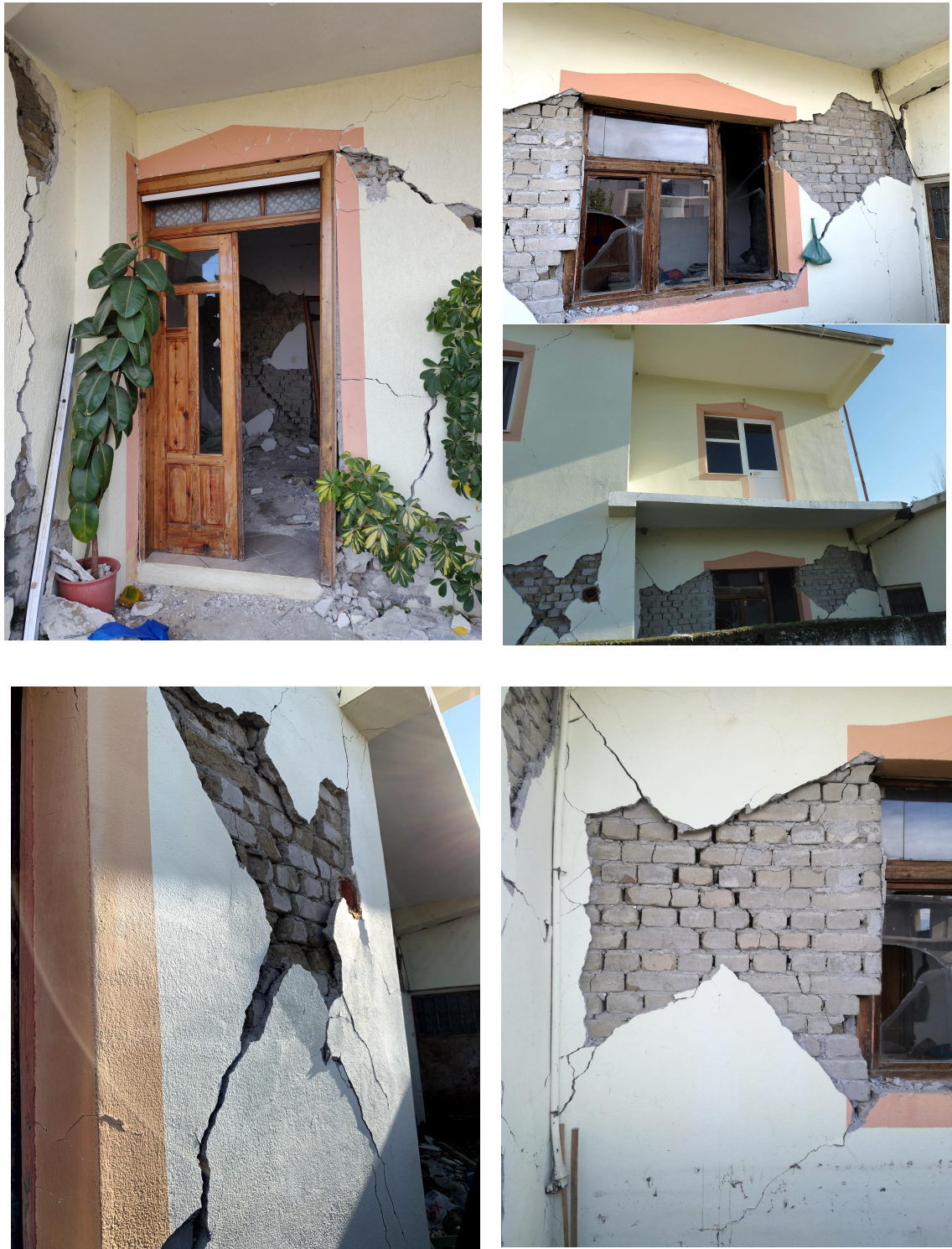
Figure 32: Major damage of three-storey confined masonry building in Thumanë.
