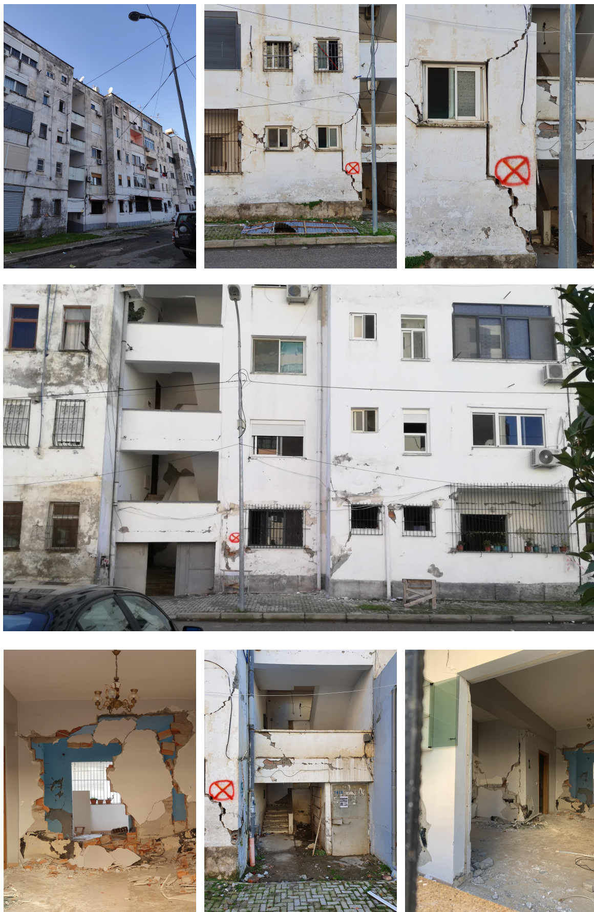
Figure 18: Major damage of 5-storey building.
