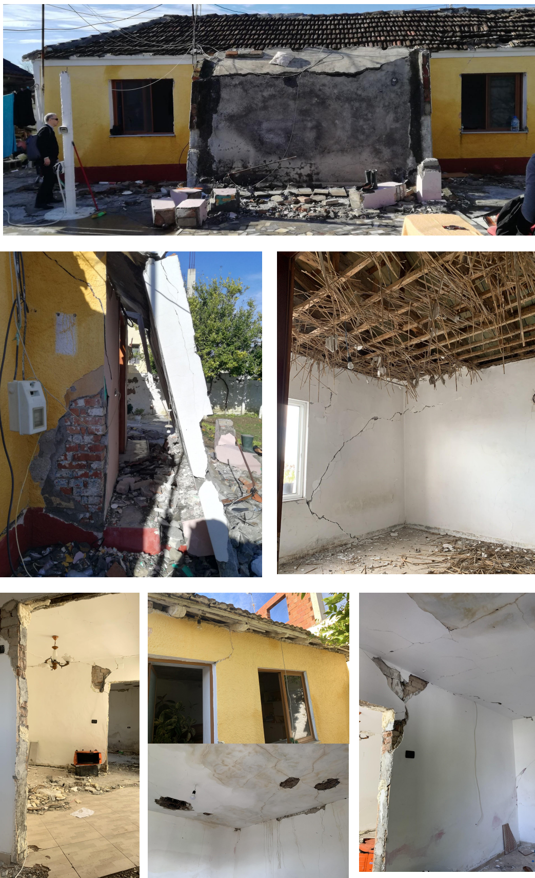
Figure 34: Major damage of single-storey building in Thumanë
