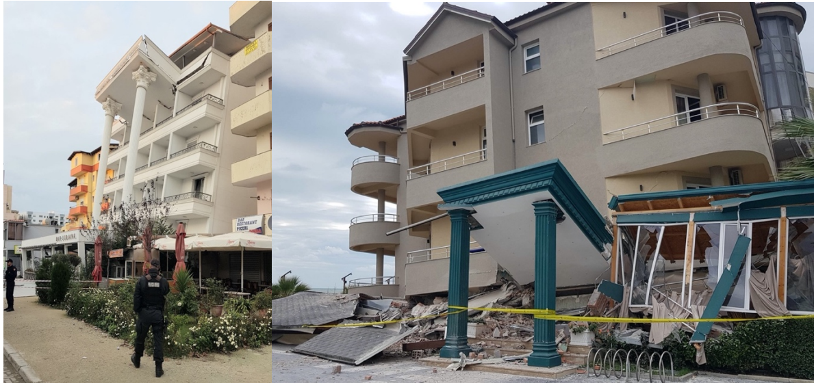
Figure 46: Tilting of Hotel Lubjana due to soil liquefaction and resulting settlement (left). Collapse of the Villa Verde Beach Hotel (photos courtesy of J. Psaropoulos)
