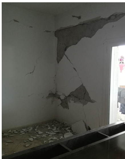
Figure 36: Major damage of two-storey RC building in Thumanë
