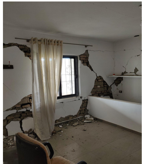
Figure 35: Moderate damage of two-storey masonry building with stone bricks, extended in plan with RC frames in Thumanë.
