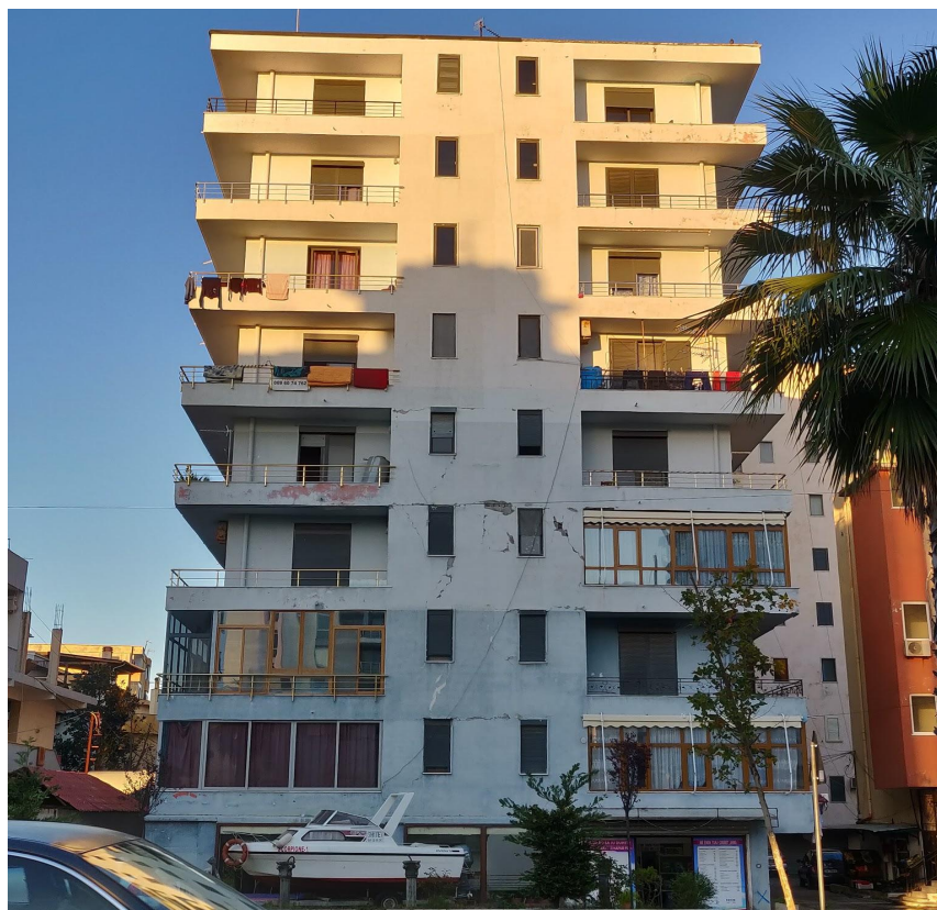
Figure 13. Light damage of an 8-storey RC building
