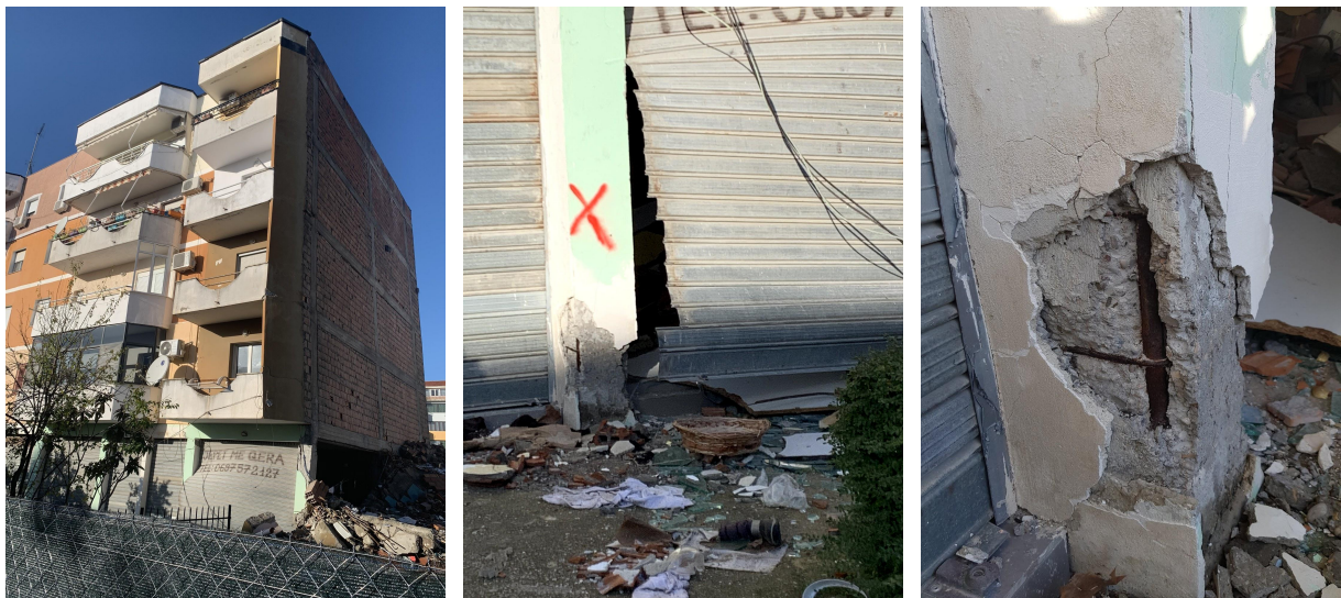
Figure 17: Major damage of 4-storey RC building
