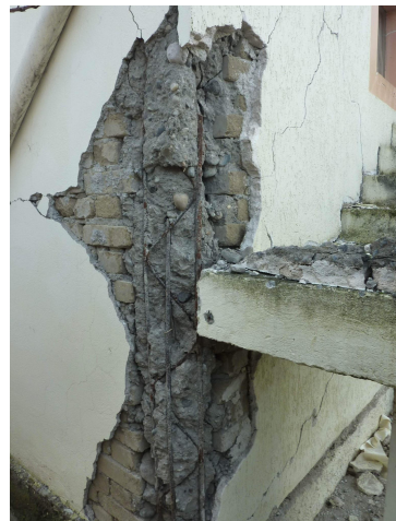
Figure 31: Major damage of three-storey confined masonry building in Thumanë.
