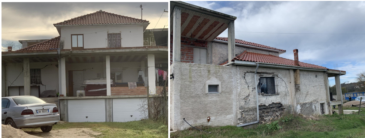
Figure 35: Moderate damage of two-storey masonry building with stone bricks, extended in plan with RC frames in Thumanë.
