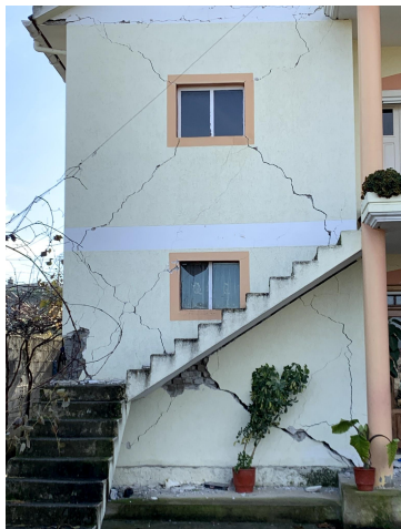
Figure 31: Major damage of three-storey confined masonry building in Thumanë.
