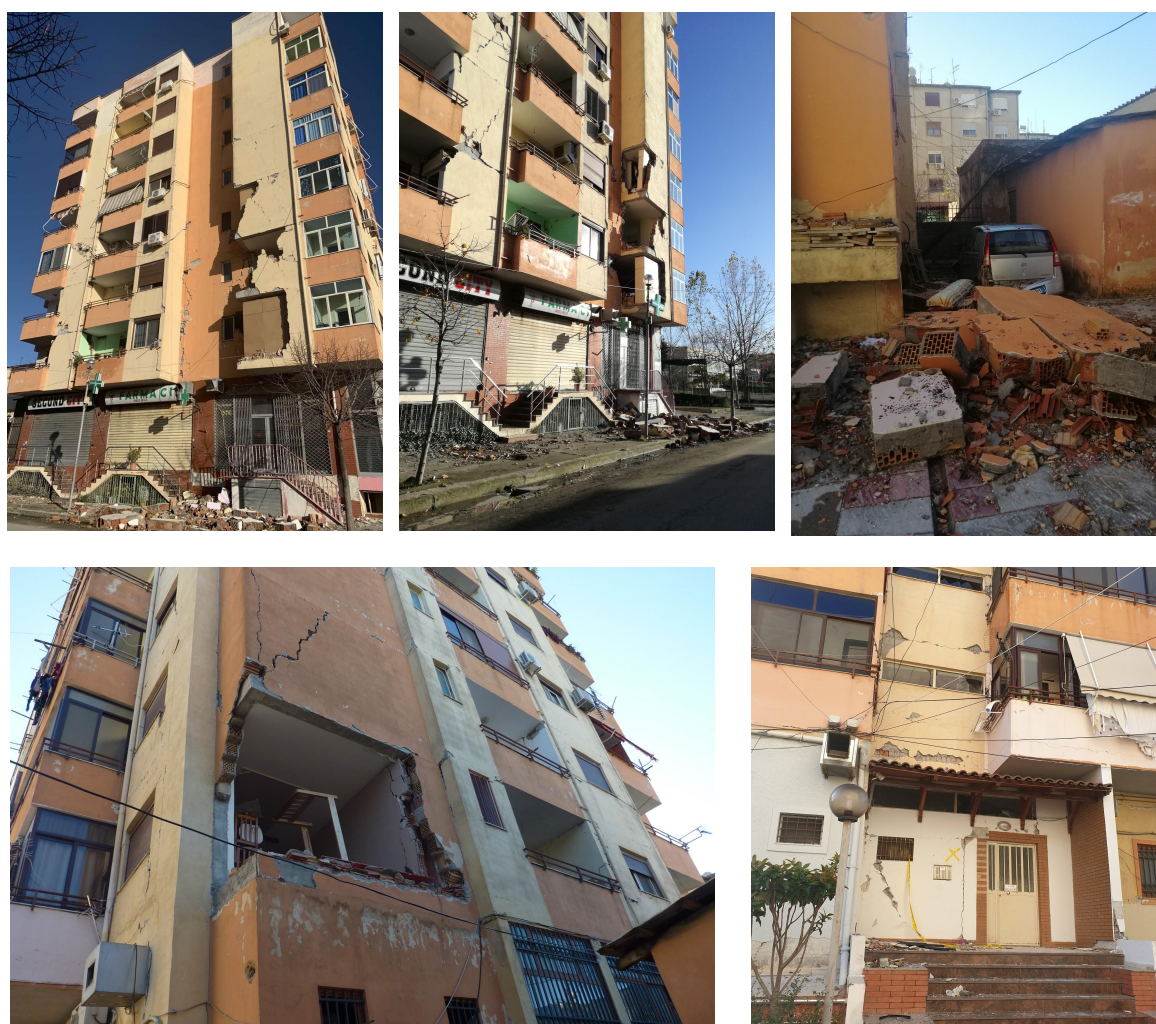
Figure 16: Major damage of an 8-storey RC building
