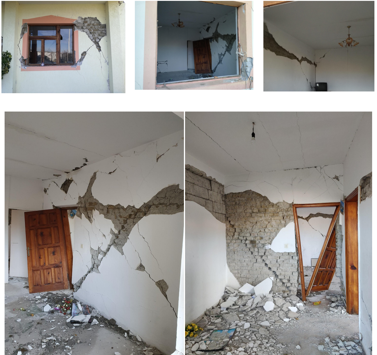
Figure 33: Major damage of three-storey confined masonry building in Thumanë.
