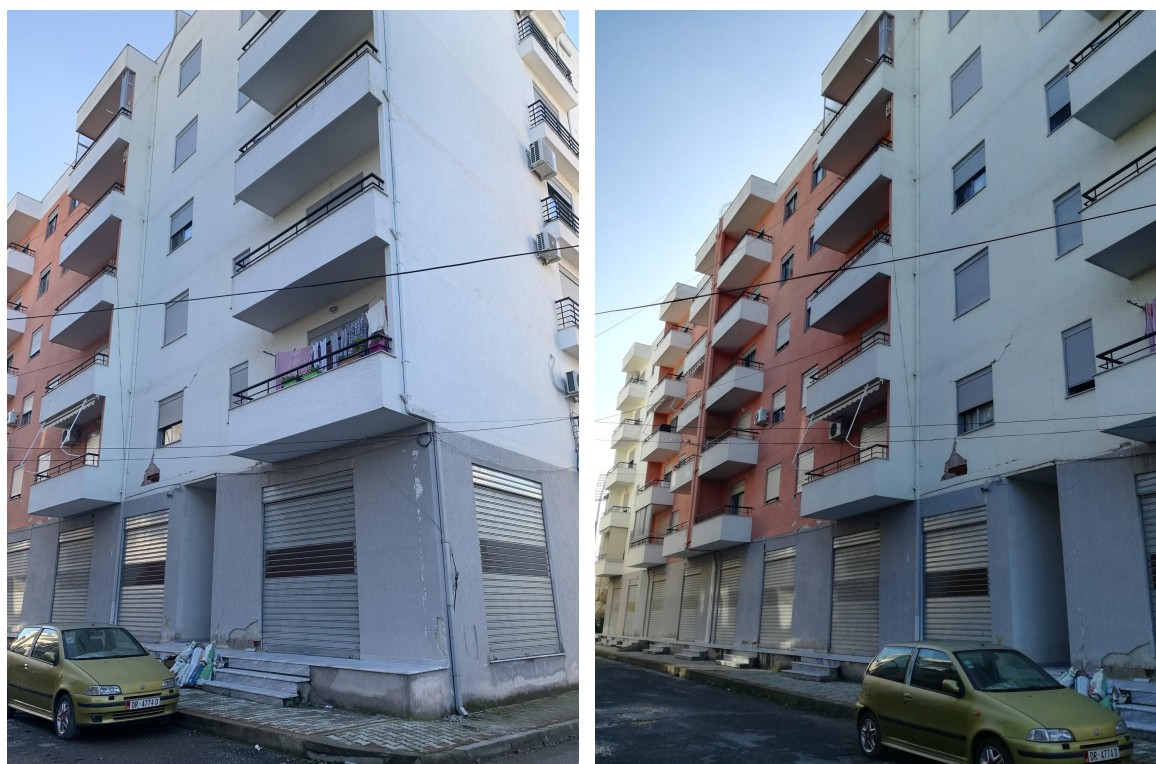
Figure 14. Moderate damage of a 5-storey RC building
