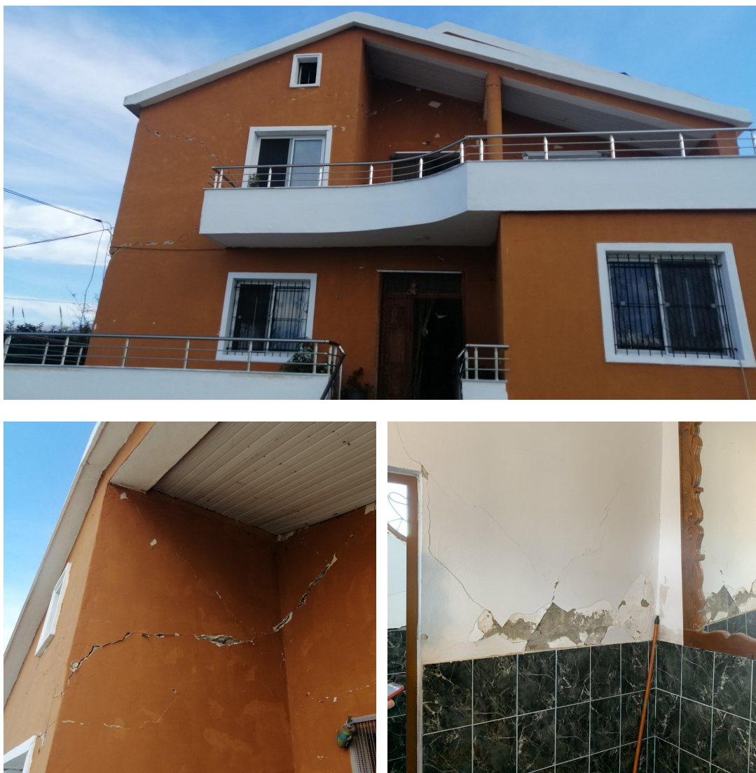
Figure 29: Moderate damage of two-storey building in Thumanë
