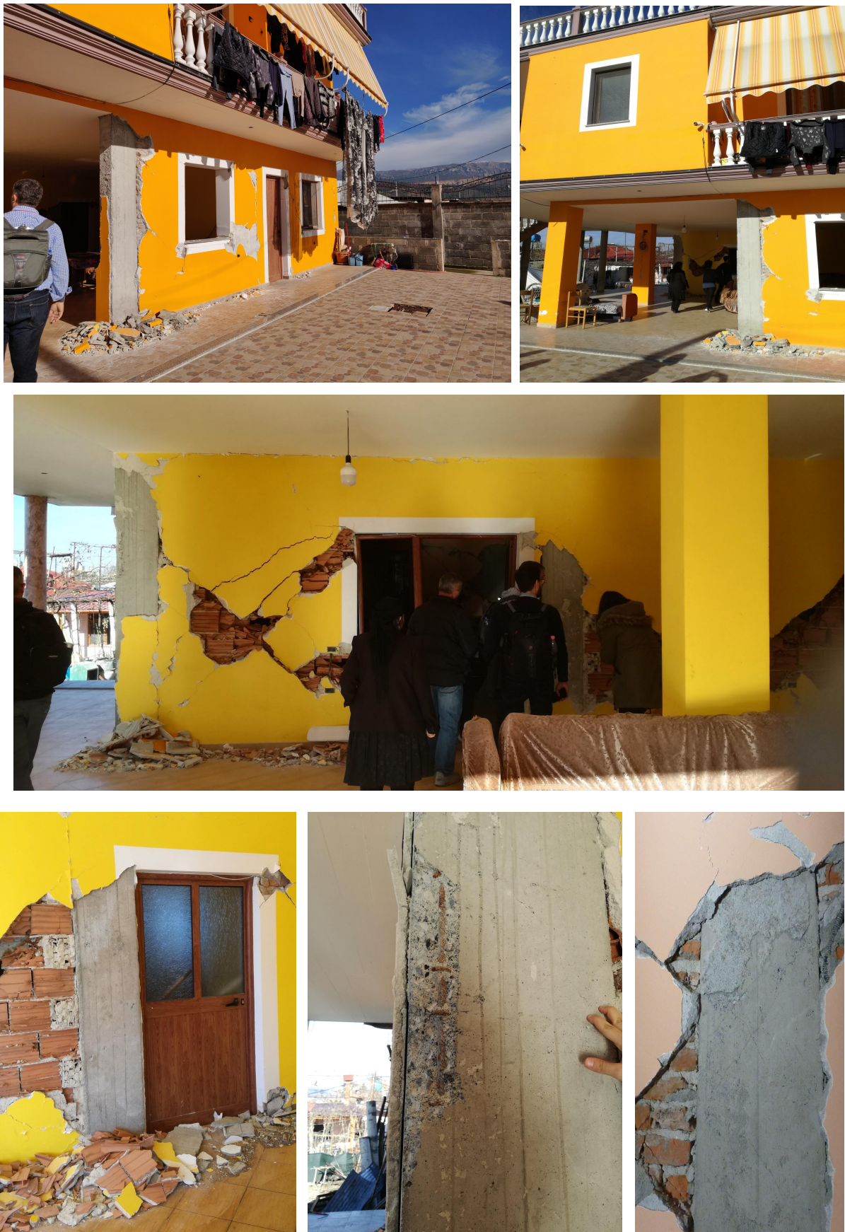
Figure 39: Major damage in the infill brick walls of a two-storey building in Thumanë.
