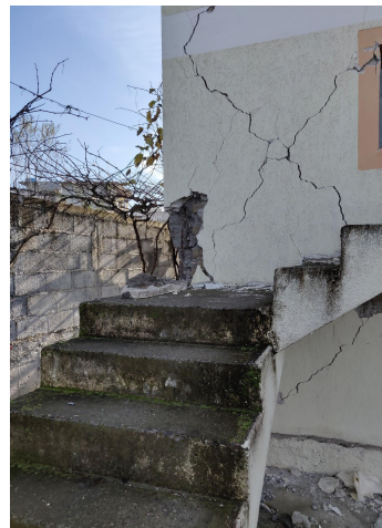
Figure 31: Major damage of three-storey confined masonry building in Thumanë.
