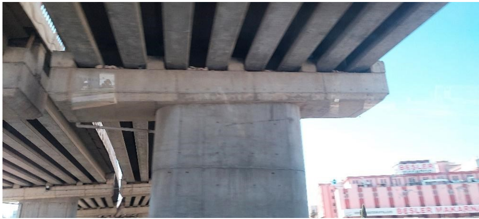
Figure 6.3 Simply supported, isolated RC bridge (overpass) in Gaziantep.
