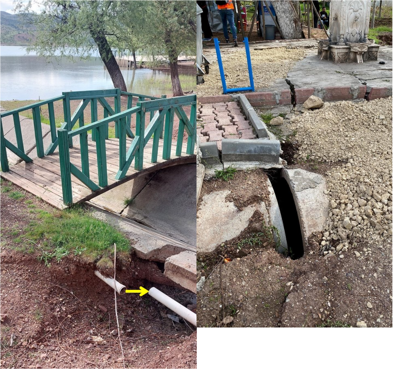
Figure 3.27 Lateral translation of the pipes at their joints because of lateral spreading close to Lake Gölbaşı (37.798226N, 37.662083E)
