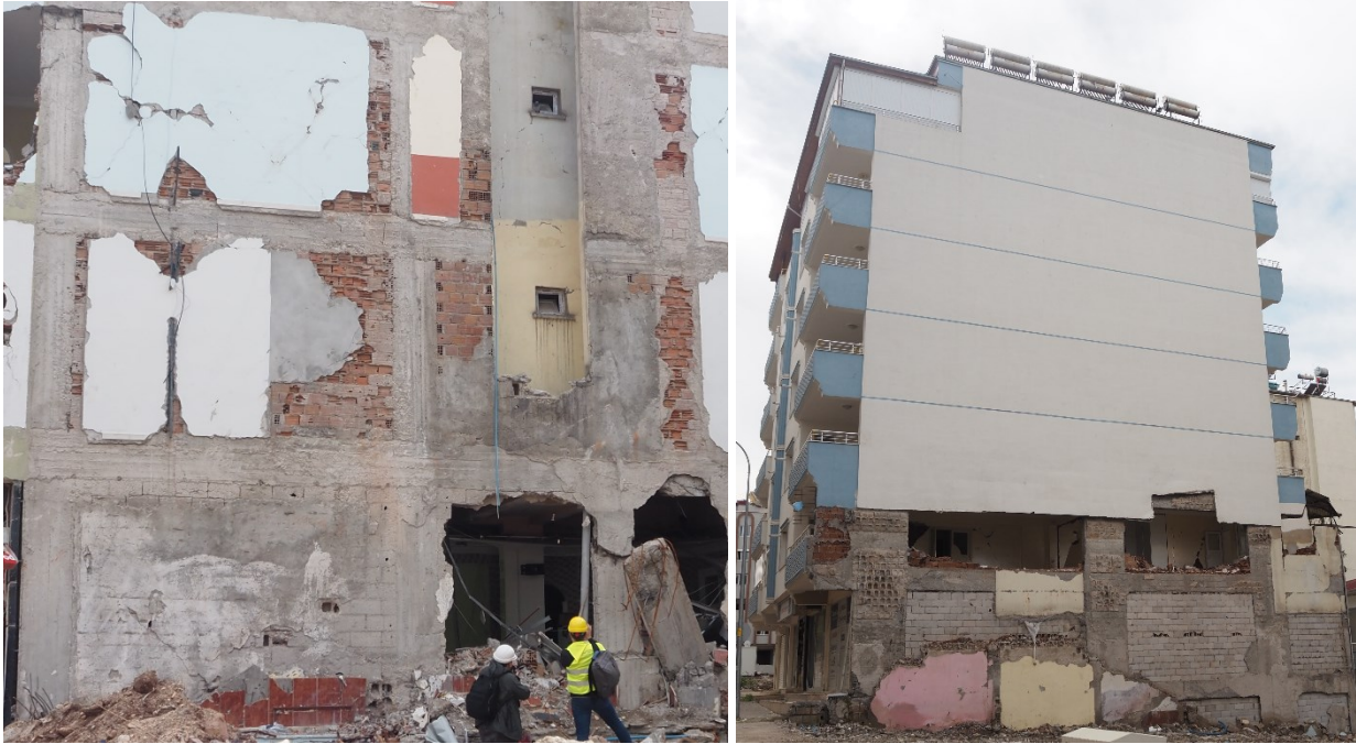
Figure 5.4.3 Infill walls made of concrete units in the ground floor, and clay brick units in the upper floors.
