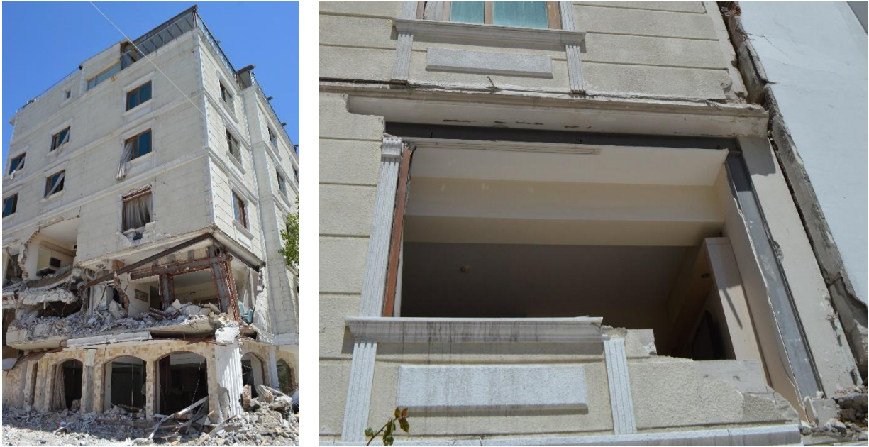
Figure 5.2.9 Concrete building was retrofitted with steel elements before the event (Antakya).
