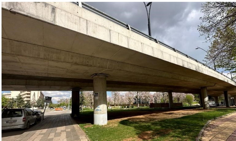
Figure 6.3 Simply supported, isolated RC bridge (overpass) in Gaziantep.
