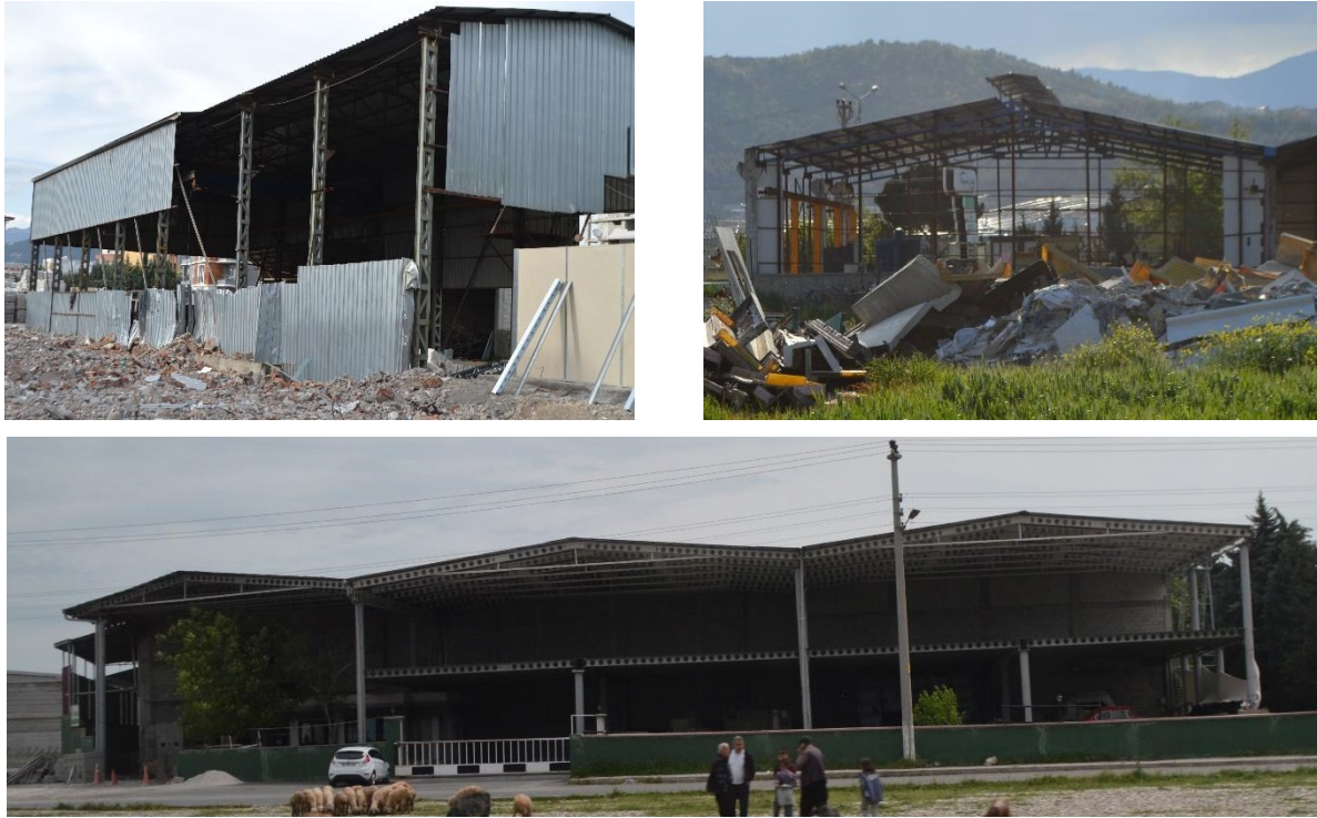
Figure 5.3.4 Structural steel industrial buildings in Adiyaman (top left) and Kahramanmaraş.
