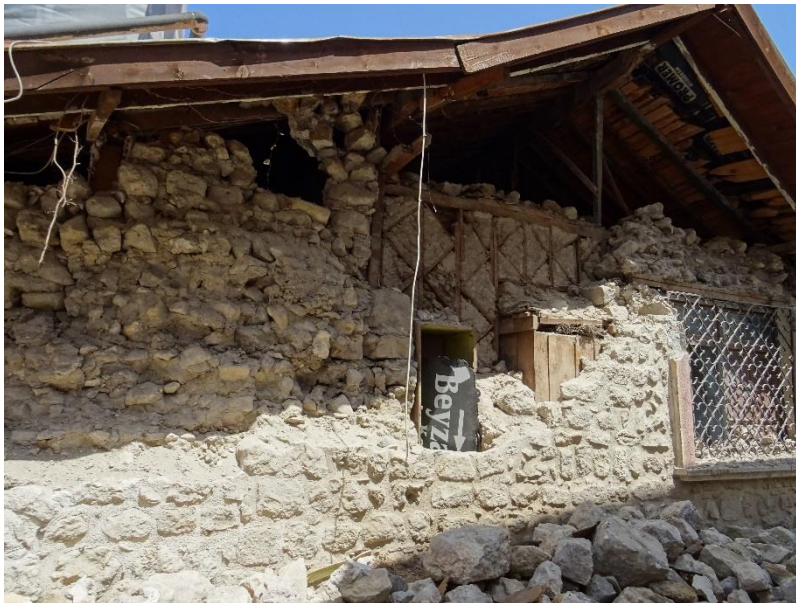
Figure 5.6.14 Antakya, three-leaf masonry with the interior leaf made of timber-framed masonry
