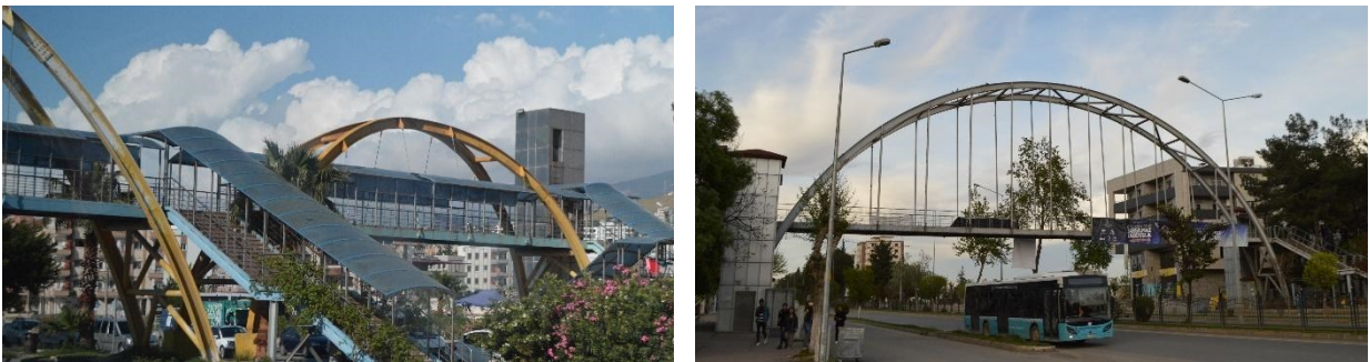
Figure 5.2.14 Pedestrian steel arch bridges in normal service, Iskenderun (left) and Adiyaman (right).
