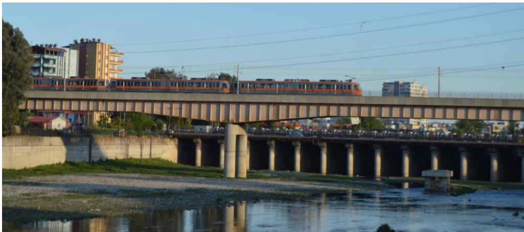
Figure 6.10 Railway bridge with steel deck in normal service
