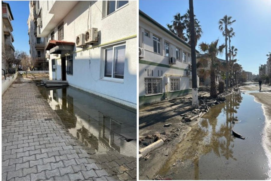
Figure 3.19 Coastal deposits from mainly composed of loose sandy deposits. The coastal zone is still flooded due to significant settlement and liquefaction phenomena.
