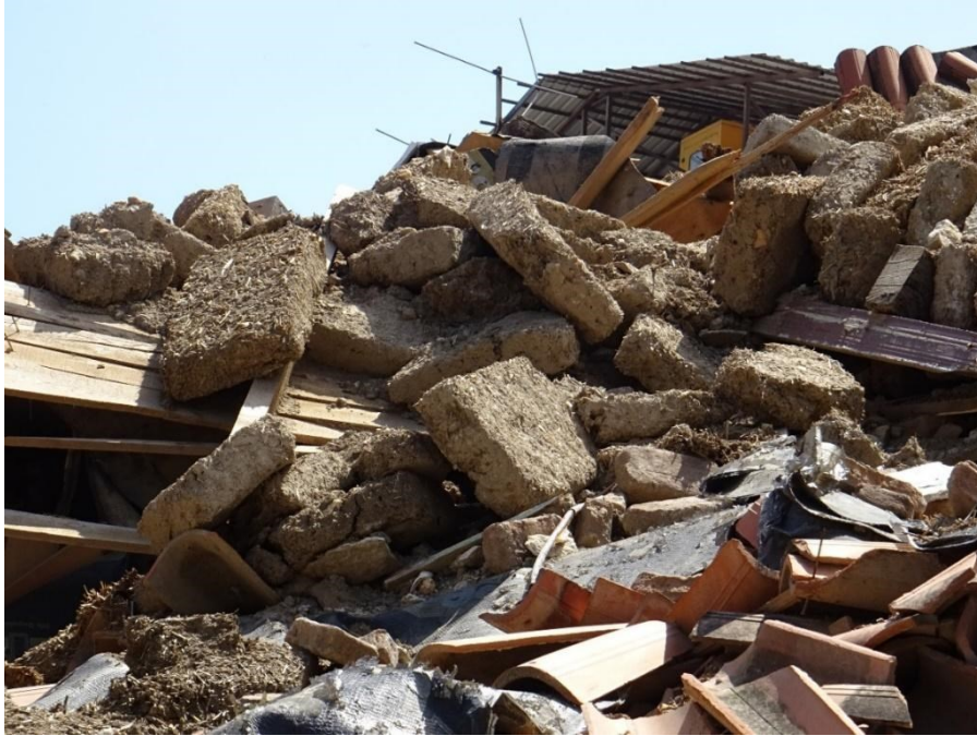
Figure 5.6.7 Antakya, collapsed building, partly made of adobe containing straw.
