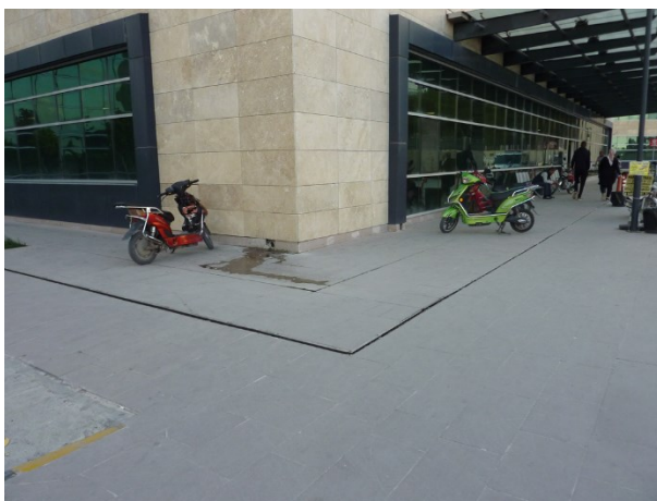
Figure 5.5.7 Dört Yol State Hospital (a) seismic joint, (b) slightly damaged tiles at the seismic joint
