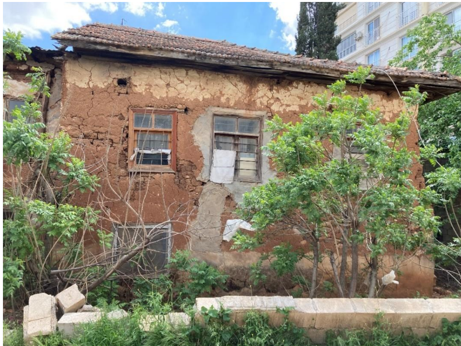
Figure 5.6.8 Islahiye, adobe building.
