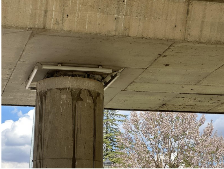
Figure 6.4 Continuous, seismically isolated RC bridge (overpass) in Gaziantep.
