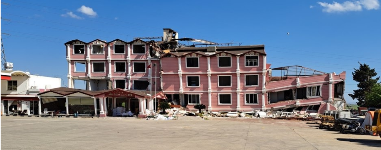
Figure 5.1.3 Collapse of soft ground story (Belen-Hatay). Photo: M.Moretti.
