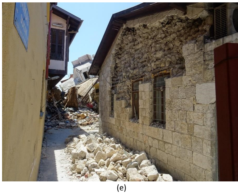
Figure 5.6.12 Antakya, stone masonry in buildings of the historical centre
