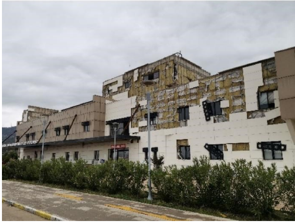
Figure 5.5.12 Nonstructural damage to the fixed-base building F2 of the Nurdağı State Hospital (a) Façade (b) damaged suspended ceiling (Credits: Qu et al.)
