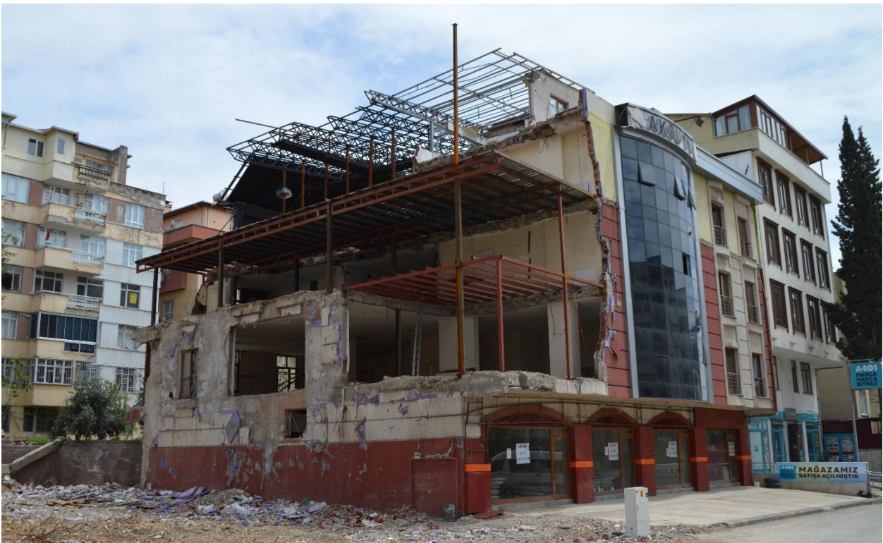
Figure 5.2.10 Restoration of concrete buildings with steel frames (Kahramanmaraş).
