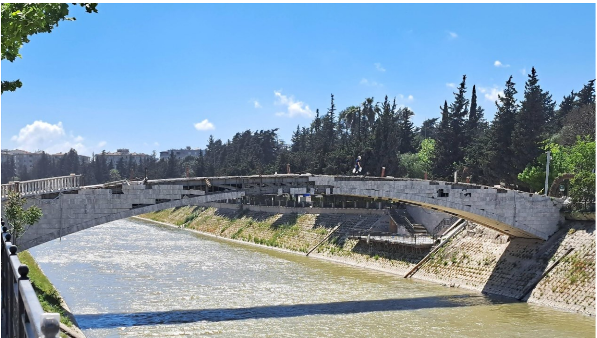
Figure 6.8 Steel truss pedestrian bridge at Antakya
