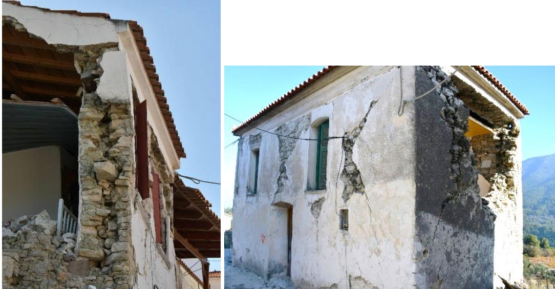
Figure 5.6.13 Samos island, typical masonry typology (2020, Samos earthquake)
