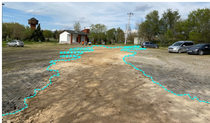
Figure 3.23 Soil ejecta at the surface, as evidence of seismic liquefaction, occurred in Gölbaşı (37.798553N, 37.662833E).
