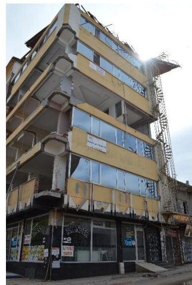
Figure 5.2.4 Top floor roof on a 6-story building in Pazarcık. Total collapse due to poor anchorage.
