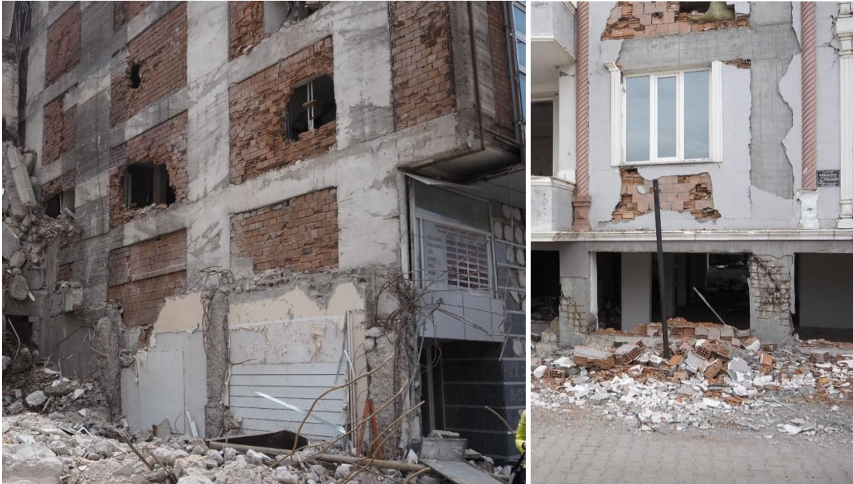
Figure 5.4.1 Infill walls made of clay bricks, of different sizes.
