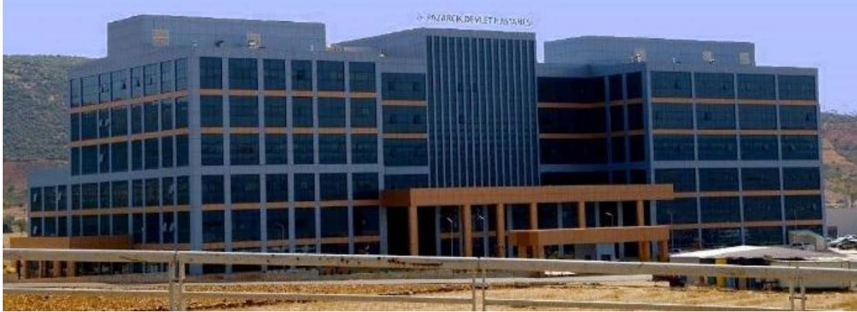
Figure 5.5.10 The conventional (non-seismic isolated) Pazarcık State Hospital (photo credits: google maps)
