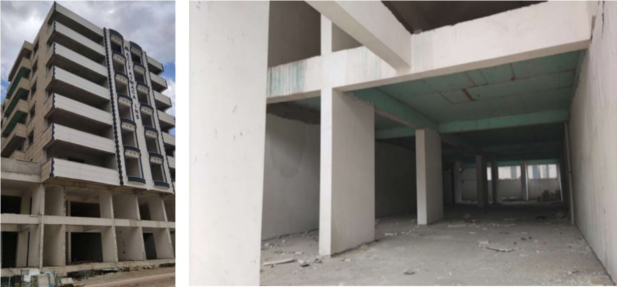
Figure 5.1.8 Building with RC shear walls in Islahiye with no apparent structural damage (constructed later than 08/2020 (source Google Earth) close to seriously damaged buildings. Photo: A.Papachristidis.
