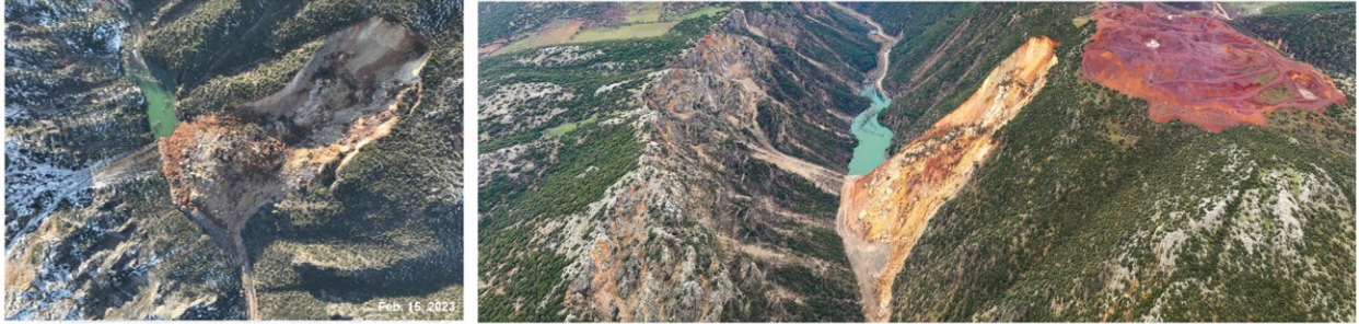
Figure 3.48 A deep-seated landslide was identified in the Islahiye region, where millions of m 3 have slid and blocked the river creating a dam behind the fallen mass.
