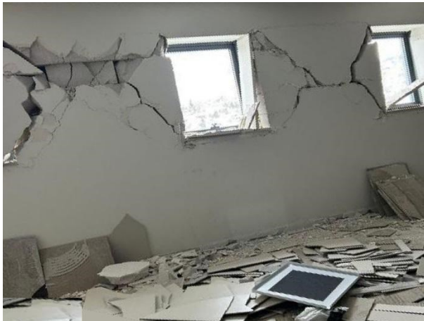
Figure 5.5.11 Pazarcık State Hospital (a), (b) heavy damage to the infill walls, suspended ceiling and EM equipment (photo credits: Sumer et al.)
