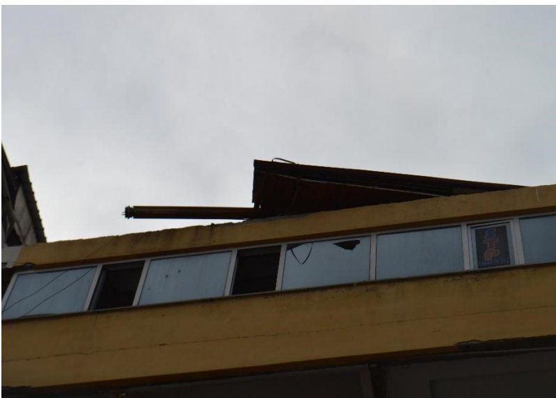
Figure 5.2.4 Top floor roof on a 6-story building in Pazarcık. Total collapse due to poor anchorage.
