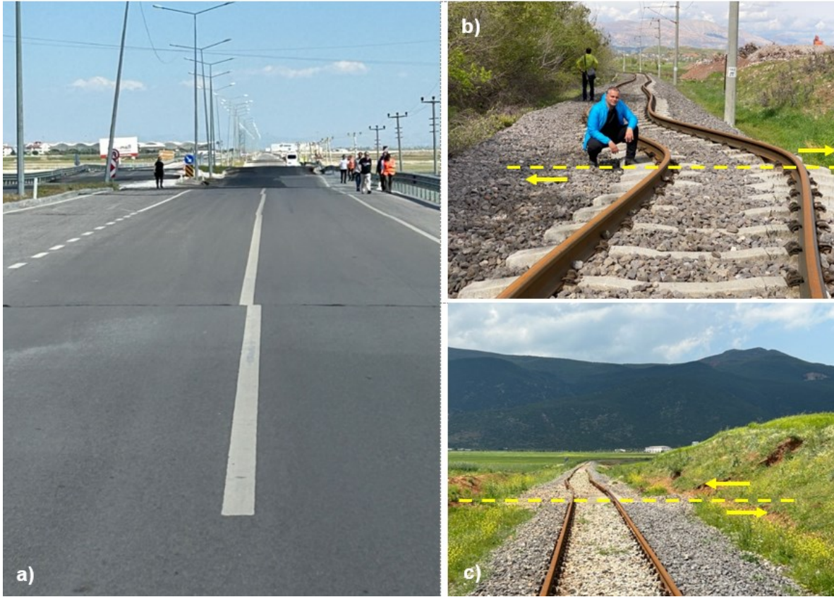
Figure 3.5 Surface ruptures in a) Antioch Airport area, b) Gulbasi c) Osmaniye.
