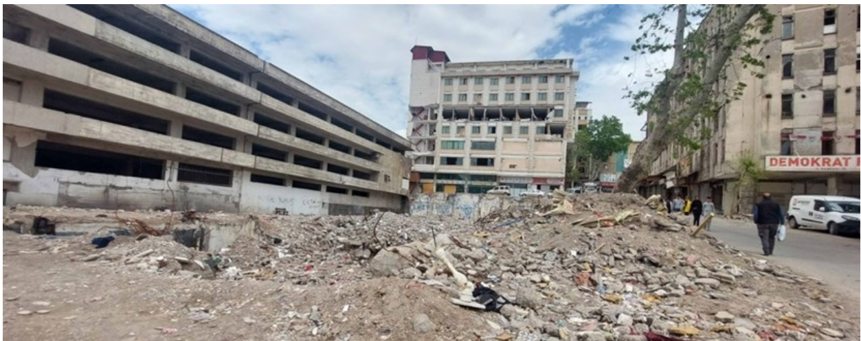
Figure 5.1.14 Building with short columns in a row which, apparently, did not suffer any damage. Photo: E.Garini.
