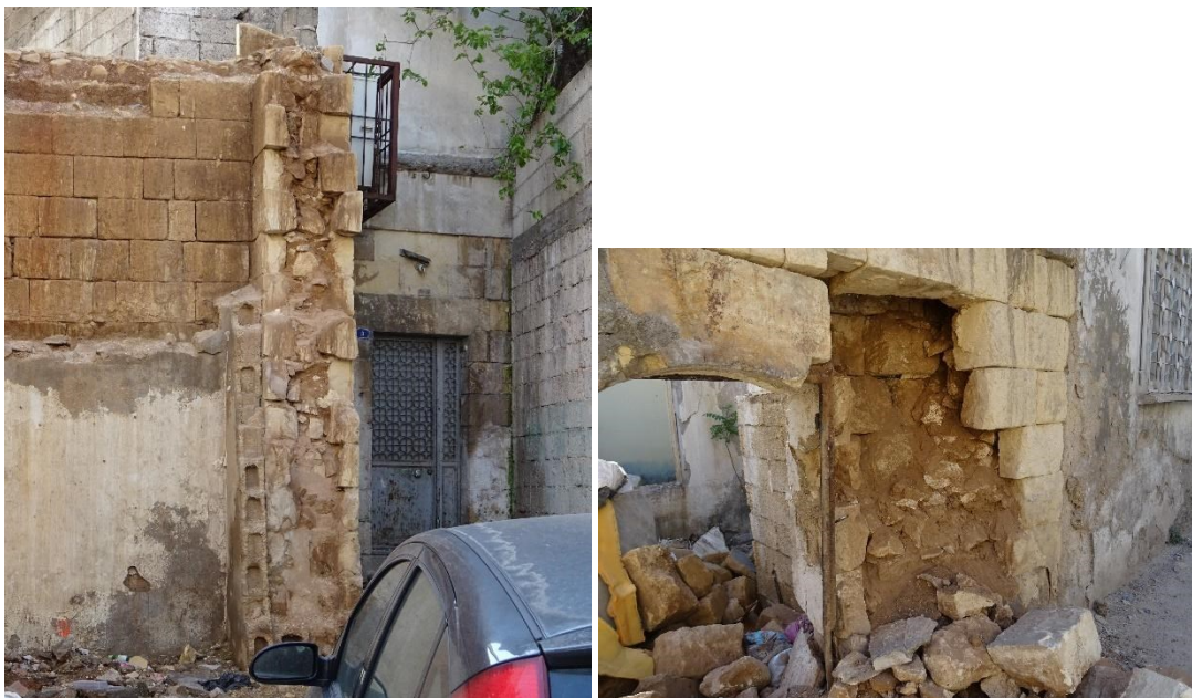
Figure 5.6.10 Gaziantep, masonry typology of a historical building
