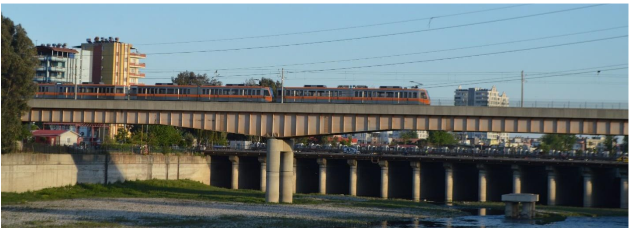
Figure 5.2.15 Railway steel bridge in normal service (Adana).
