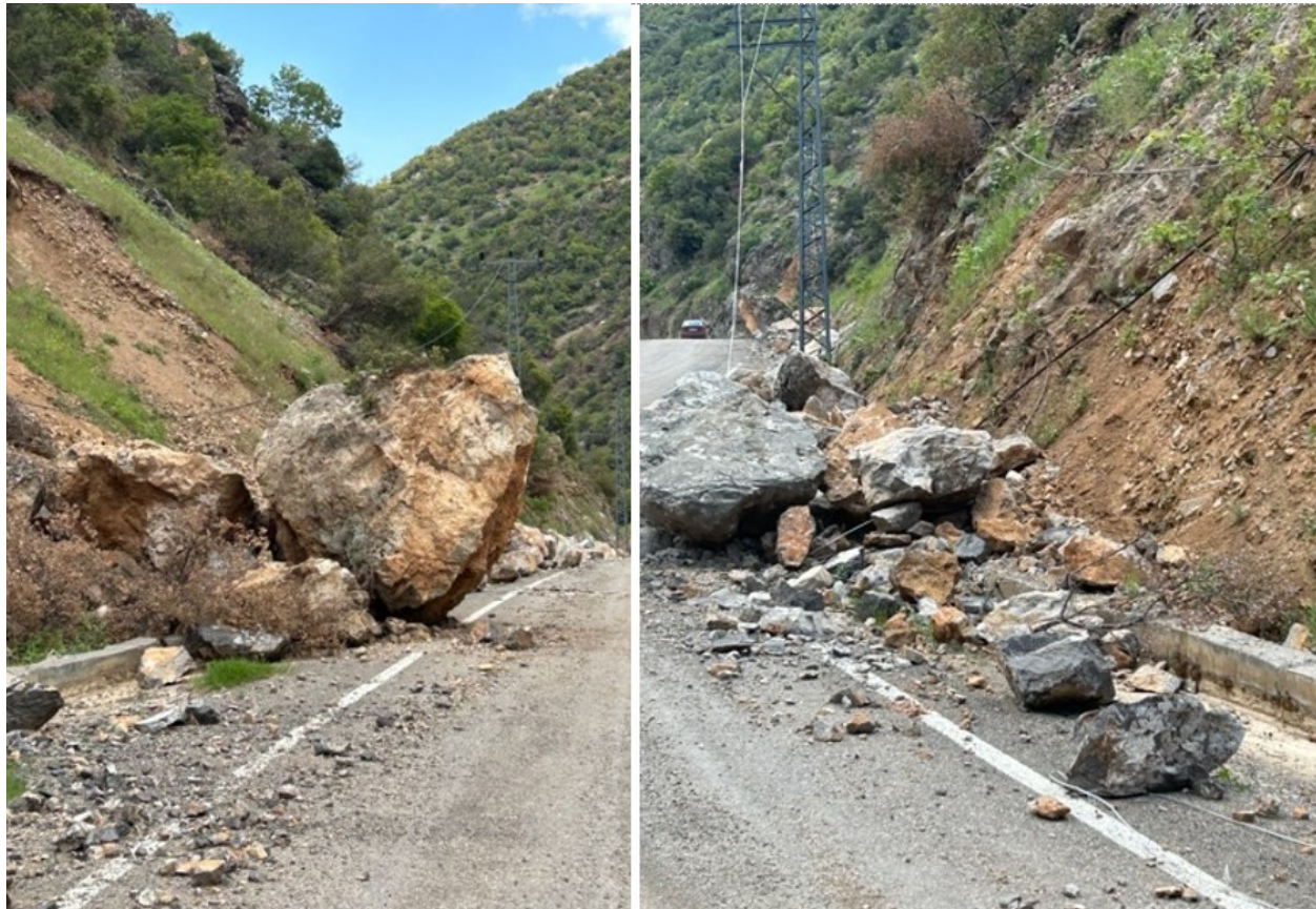
Figure 3.47 Rockfall incidents in the Islayie region in limestone steep terrain close to Islahiyi area. Blocks reached up to sizes of 6-7m 3 .
