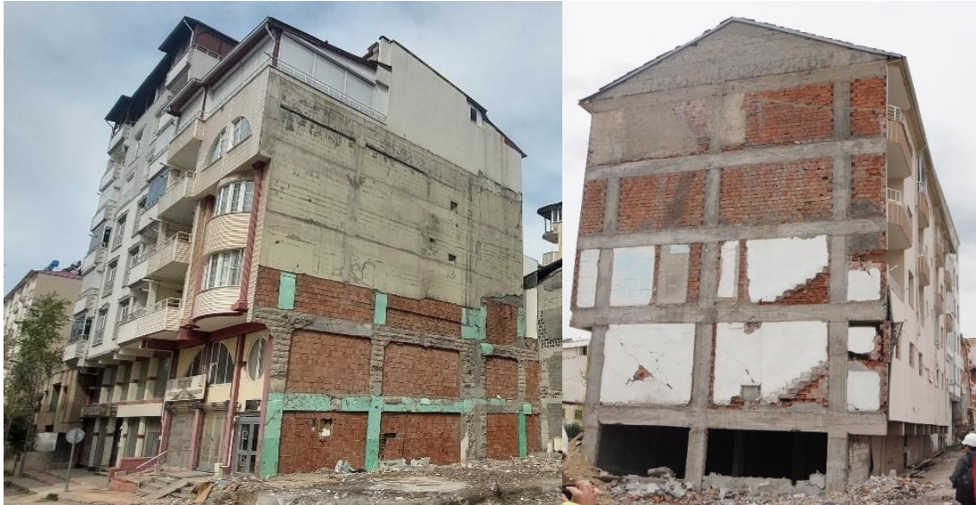
Figure 5.4.5 Walls constructed with the use of RC tie beams.
