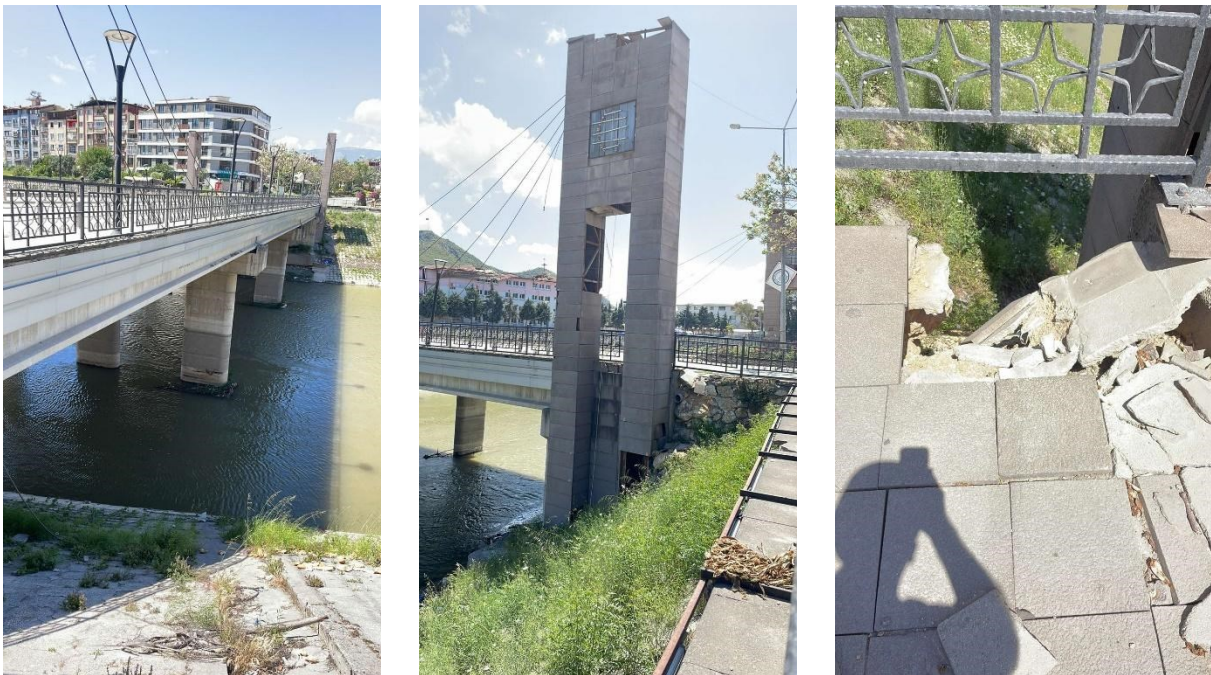
Figure 5.2.12 Road bridge with steel tower (Antakya).
