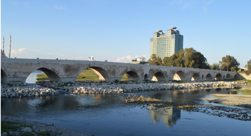
Figure 6.9 Masonry bridge in Adana
