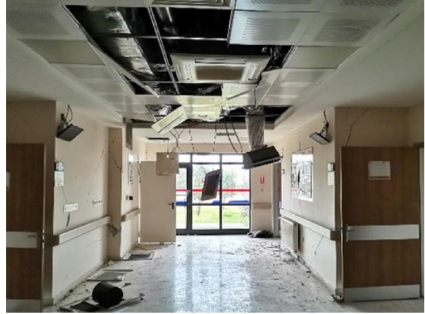
Figure 5.5.12 Nonstructural damage to the fixed-base building F2 of the Nurdağı State Hospital (a) Façade (b) damaged suspended ceiling (Credits: Qu et al.)
