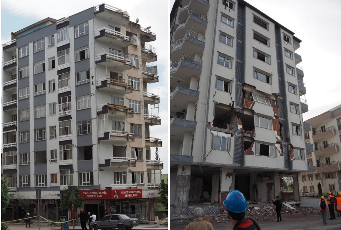
Figure 5.4.7 Overhangs, constructed upon cantilever slabs.
