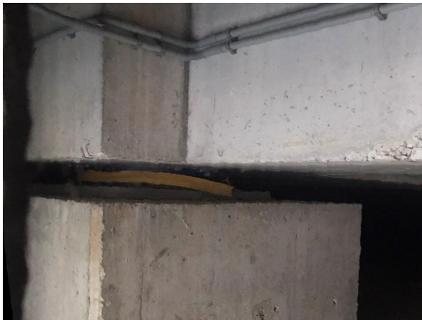
Figure 5.5.6 Dört Yol State Hospital I (a), (b) isolators layout at the basement level
