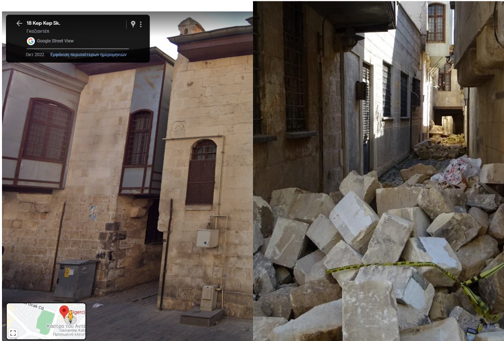
Figure 5.6.2 A street in the old part of Gaziantep, before (source: Google maps, street view, October 2022) and after the February 2023 earthquakes.
