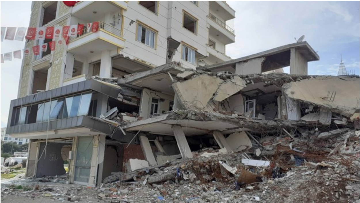
Figure 5.1.4 Collapse of RC building with flat slabs along the weak direction of the vertical structural elements (Adiyaman). Photo: E. Vougioukas.
