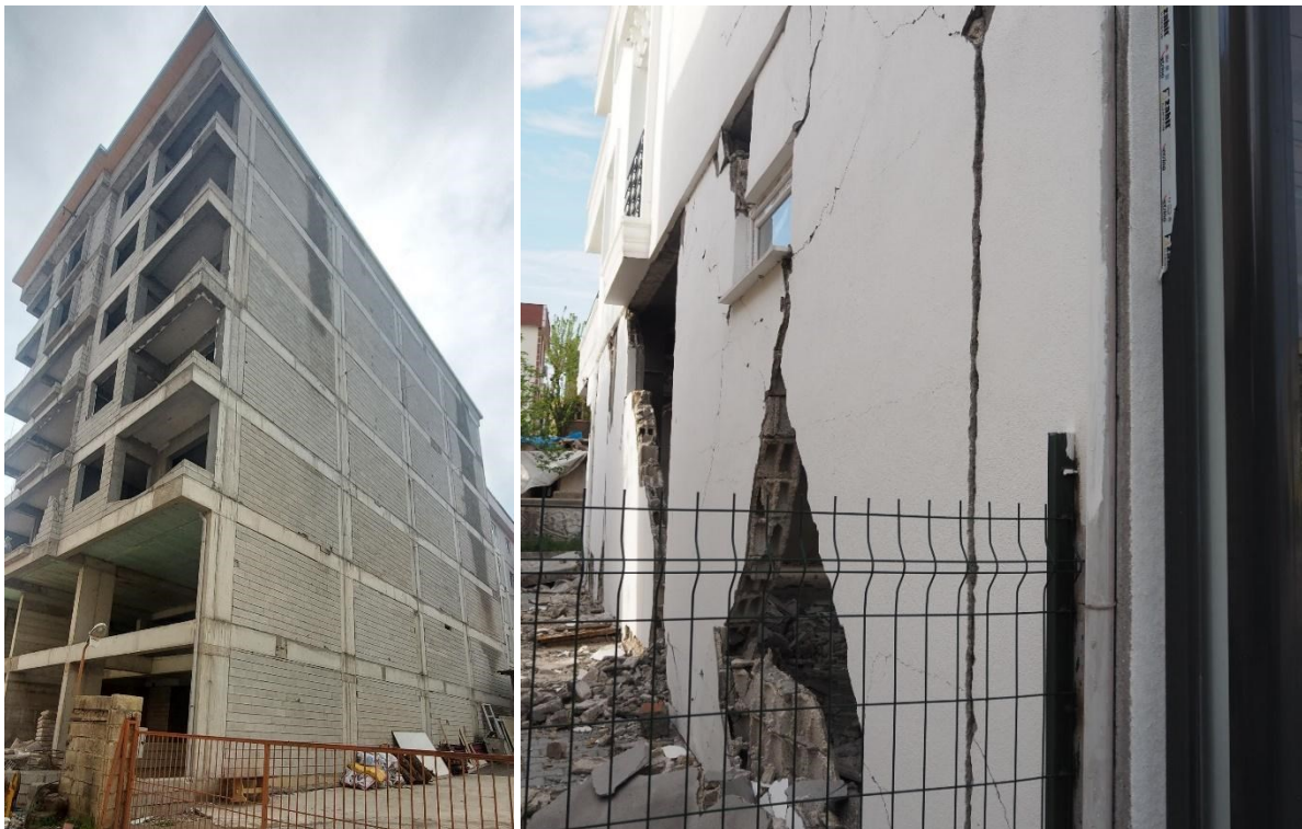
Figure 5.4.2 Infill walls made of concrete units.
