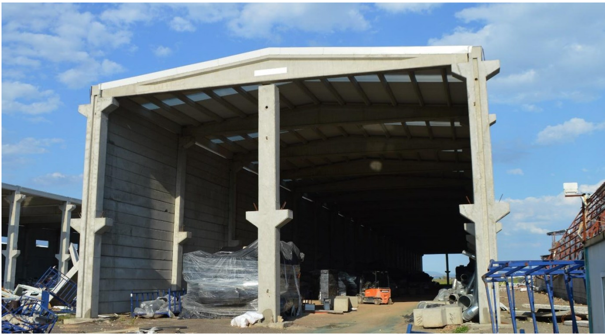
Figure 5.3.1 Typical reinforced concrete industrial building (Kahramanmaraş).
