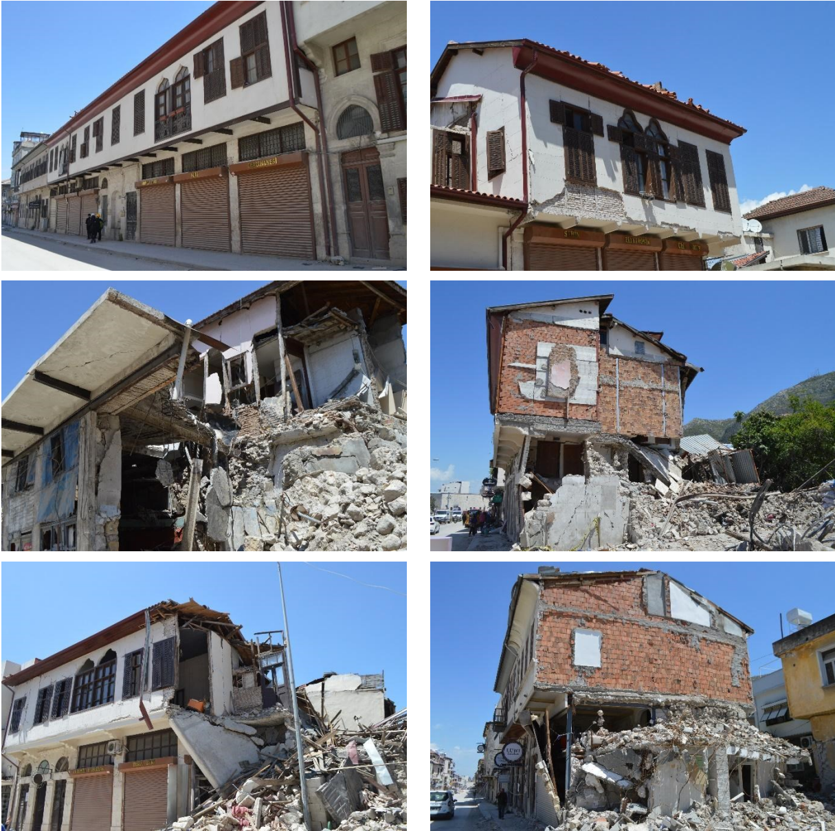
Figure 5.2.8 Various 2-story buildings along Kurtuluş Avenue in Antakya.
