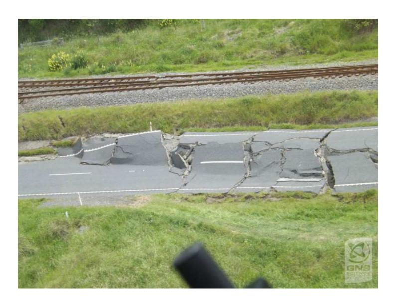
Rupture of the Hundalee Fault displacing SH1 and the railway line.
