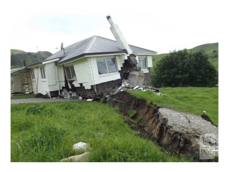
Thrust-Fault Rupture directly under the middle of a single-storey house (about 32km north-east of Kaikoura).
