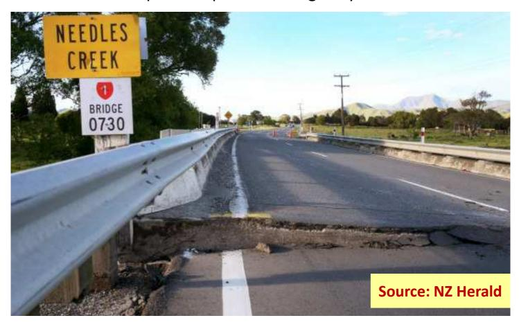
Damage to "Needles" Bridge Abutment (?) north of Ward.
